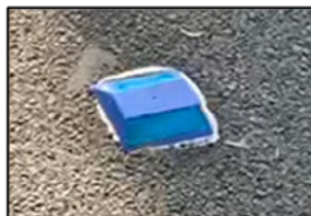
Figure 6-1 Blue Road Reflector
