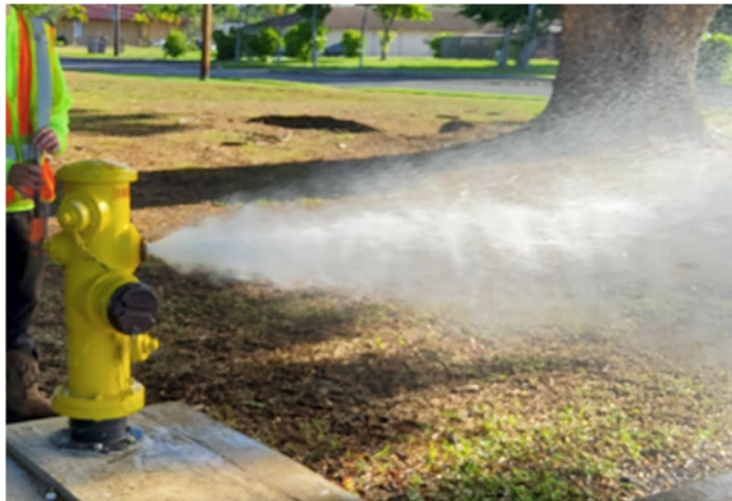
Figure 6-4 Hydrant Flushing
