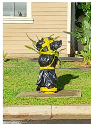
Figure 6-15 Hydrant Covered in Trash Bag
