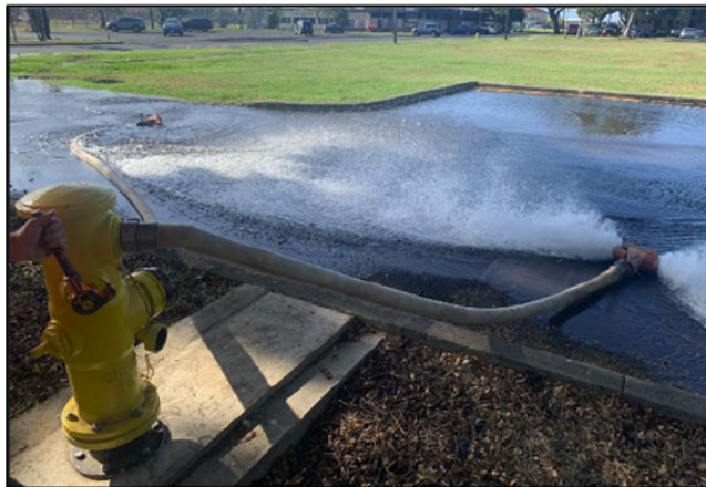
Figure 6-12 Two-Flow Hose Attachments
